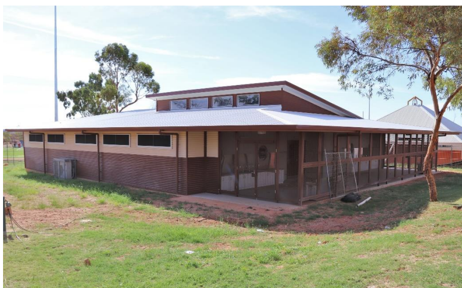
New Building: Four Classrooms and Shared Space
